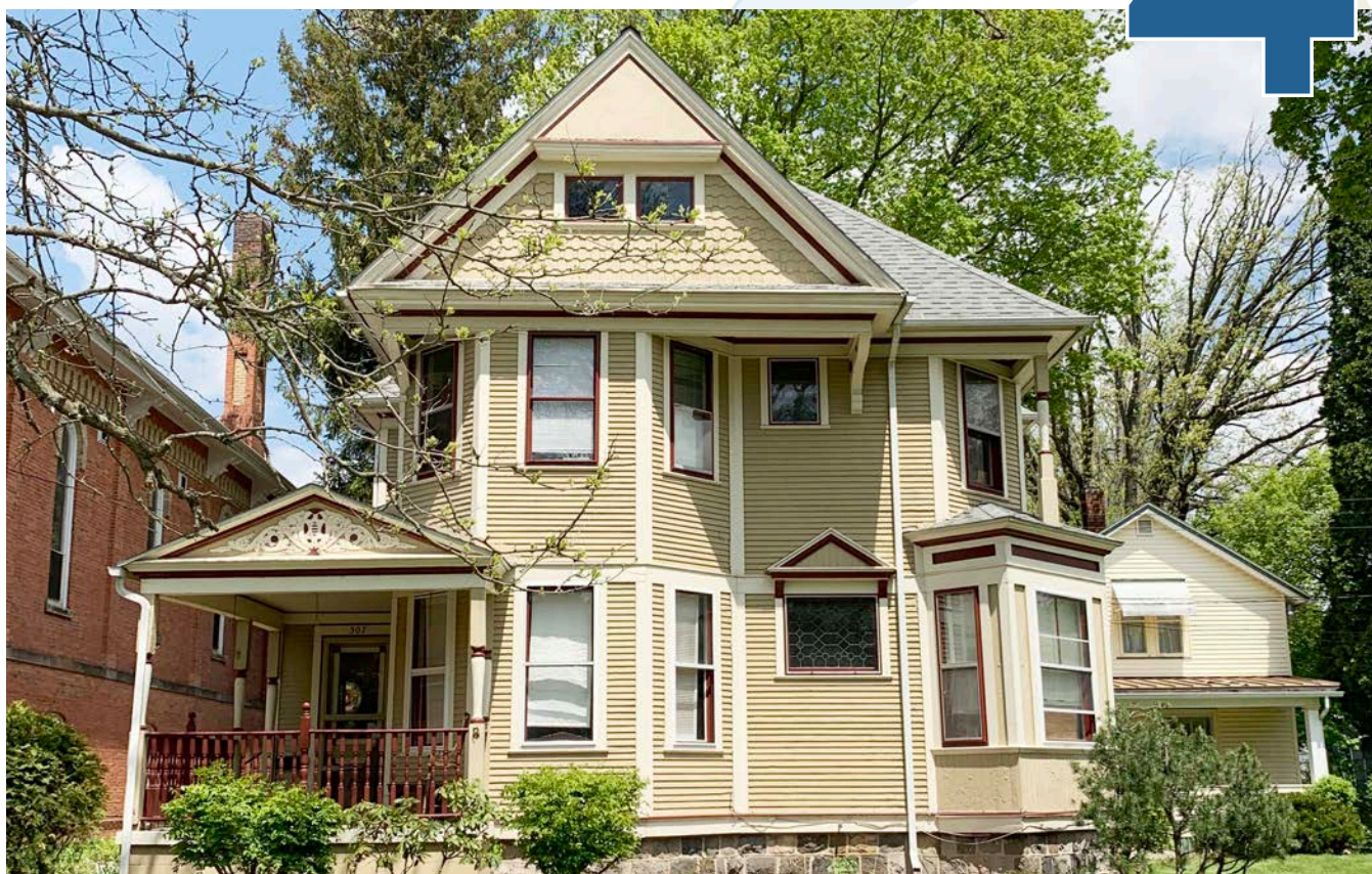
Image Source: City of Albion
