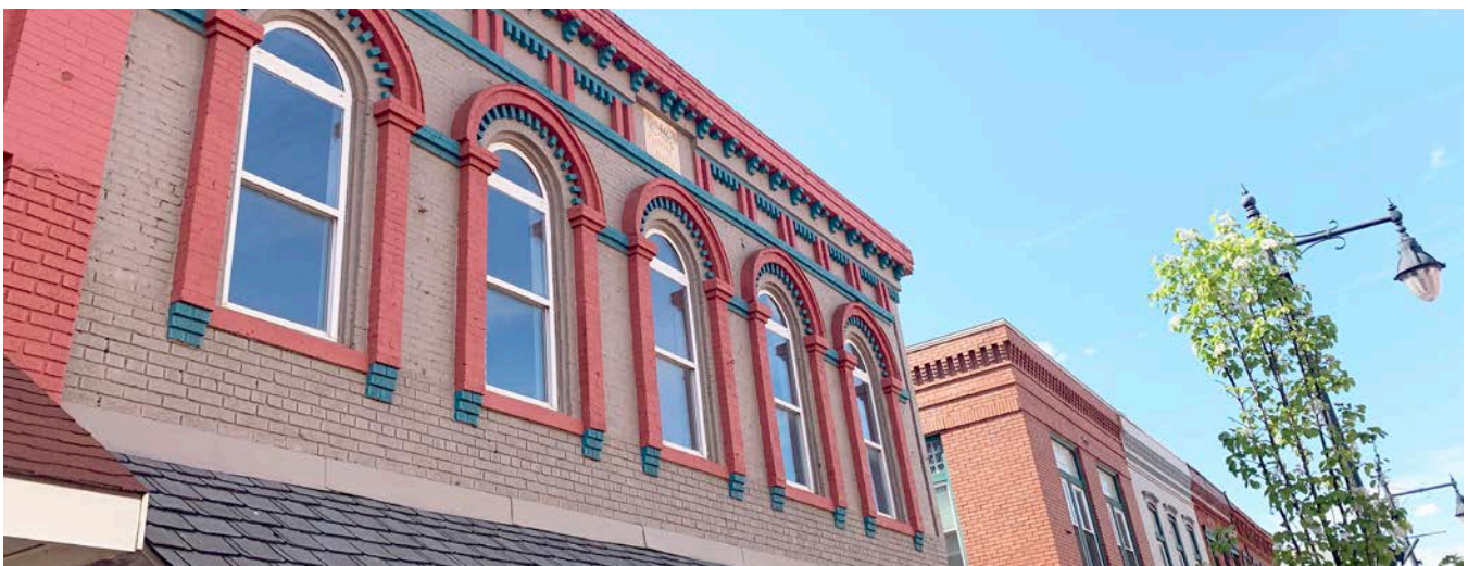
Downtown upper facades. Source: City of Albion
